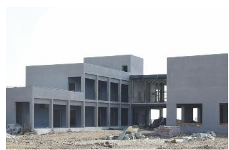
Pre-K-6 School building under construction
